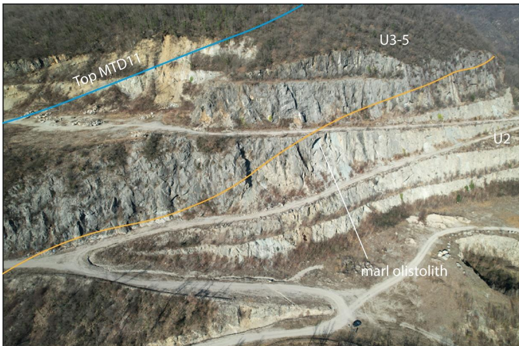
Figure 8.6 drone image of the Vernasso quarry. Focus on the MTD11.
